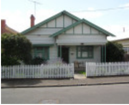
24 Potter Street, Geelong West
