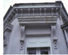
glenara glenara road bulla drawing room bay exterior dec1983
