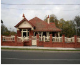
ALPHINGTON LUCERNE CRESCENT 2.jpg
