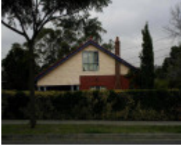
ALPHINGTON LUCERNE CRESCENT 34.jpg
