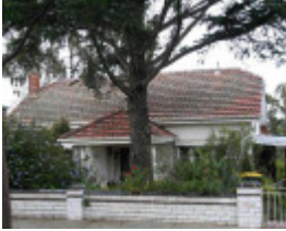
ALPHINGTON LUCERNE CRESCENT 36.jpg
