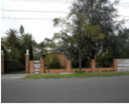
ALPHINGTON LUCERNE CRESCENT 50.jpg
