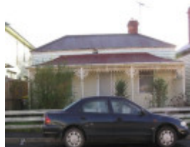
44 Preston Street, Geelong West
