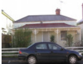
44 Preston Street, Geelong West
