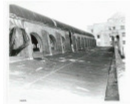
Mining Exchange_Roof_2_1976 Source: Private collection
