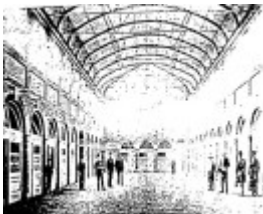
Mining Exchange04 - Mining Exchange interior shortly after opening (the date '1887' has been written on the original photo; obviously erroneous) This view clearly show the layout of the booths and their original joinery - Ballarat Conservation Study, 1978
