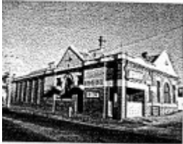
Offices Sunnyside Mills - Ballarat Heritage Review, 1998
