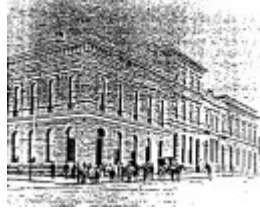
ANZ Bank03 - 'Leonard Terry Streetscape' in Lynciard Street with the former Bank of Australasia on the corner of Sturt Street - Ref: H1774, La Trobe Library - Ballarat Conservation Study, 1978
