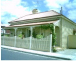
3 St James Street, Geelong West
