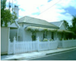
5 St James Street, Geelong West
