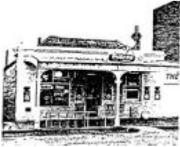
Verandahed Shop, mair Street Film 61 / Frame 38 - Ballarat Conservation Study, 1978
