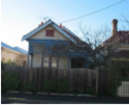
10 Tayler Street, Geelong West
