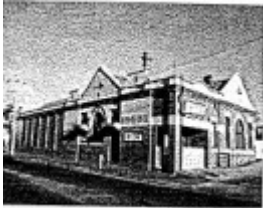
Offices Sunnyside Mills - Ballarat Heritage Review, 1998
