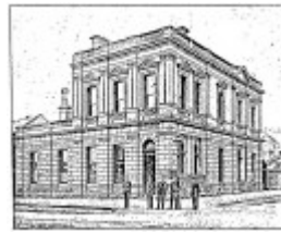
Ballarat Water Commissioners Offices02 - Ballarat Water Commissioner's Building in its original form - Ballarat Conservation Study, 1978
