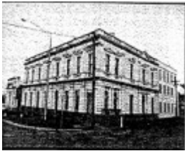
Ballarat City Council Offices - Ballarat Heritage Review, 1998
