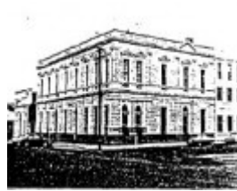
Ballarat Water Commissioners Offices - film 6 / frame 12 - Ballarat Conservation Study, 1978
