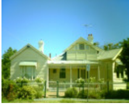
7 Villamanta Street, Geelong West
