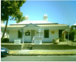
11 Villamanta Street, Geelong West
