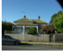
Historic photo, 29 Villmanata St - Glg West Conservation Study_resize.jpg
