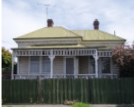
29 Villamanta St, Geelong West
