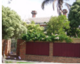
35 Villamanta St, Geelong West
