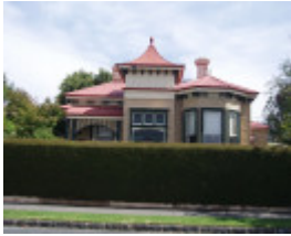
37 Villamanta St, Geelong West
