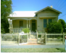
55 Villamanta Street, Geelong West
