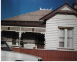
61 Waratah Street, Geelong West
