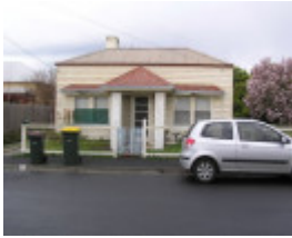
63 Waratah Street, Geelong West
