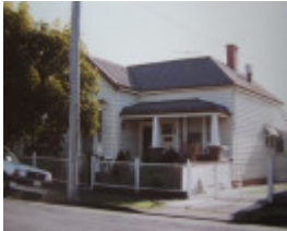
20 Waratah Street, Geelong West
