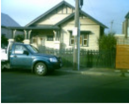
25 Waterloo Street Geelong Wes
