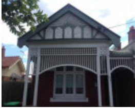
House 279 Ascot Vale Road
