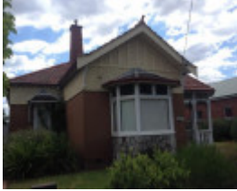
House 277 Ascot Vale Road
