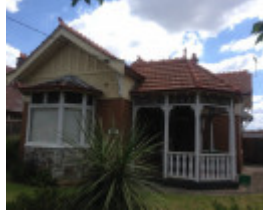
House 277 Ascot Vale Road
