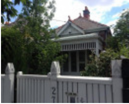
House 273 Ascot Vale Road
