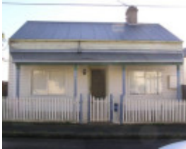
24 Weller Street, Geelong West
