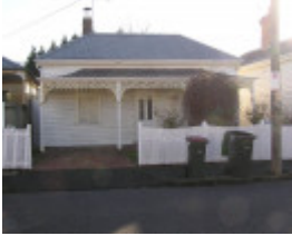
60 Weller Street, Geelong West
