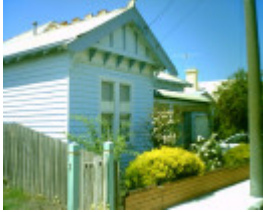
144 Weller Street, Geelong West
