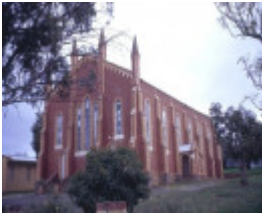
Former Wesleyan Methodist Church Elser Street California Gully Eaglehawk Right Side
