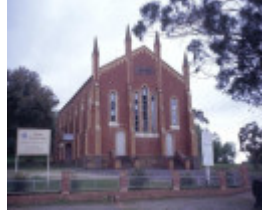
Former Wesleyan Methodist Church Elser Street California Gully Eaglehawk
