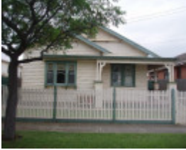
32 Anderson St, Geelong East
