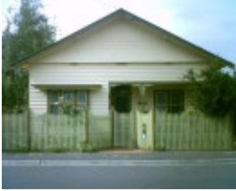
97 Waratah Street, Geelong West
