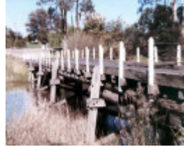
B7477 Tambo River Bridge
