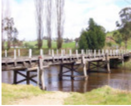
B7477 Tambo Upper Bridge
