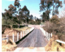
B7477 Tambo River Bridge
