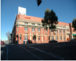
Electric Light & Trading Co - 82 Brougham Street, Geelong
