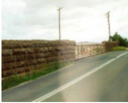
B7465 Riddells Creek Bridge
