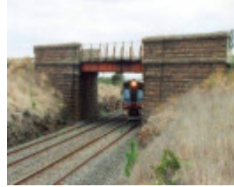
B7465 Riddells Creek Bridge
