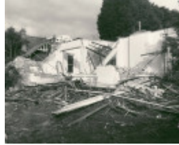
B3525 Kirn Demolished
