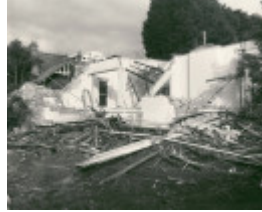
B3525 Kirn Demolished
