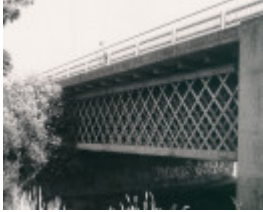
B7474 Bell Street Bridge
