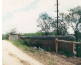
B7468 Burgoyne Street Bridge
