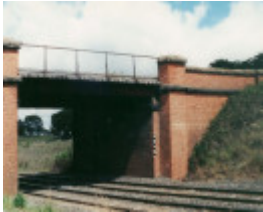
B7468 Burgoyne Street Bridge
