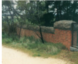
B7468 Burgoyne Street Bridge
