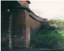
B7468 Burgoyne Street Bridge
