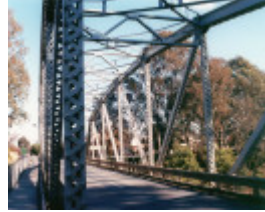
B7481 Murchison Bridge
