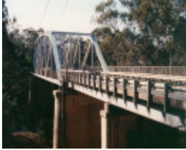
B7481 Murchison Bridge
