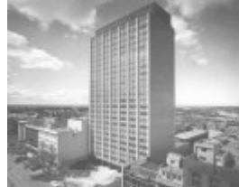
B7651 CRA Building
