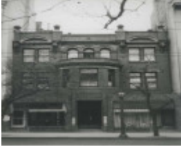
B7653 Barretts Building.jpg
