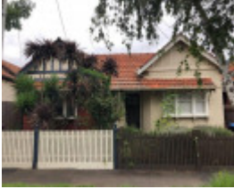
41-43 Banole Avenue, Prahran
