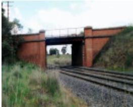
B7494 Forrest Road Bridge
