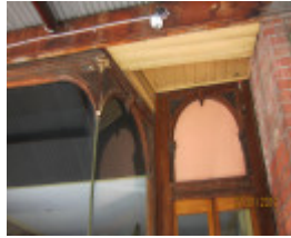
Shopfront details, 150 Lygon St
