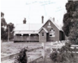
B3114 Frmr State School & Residence High St Cranbourne
