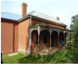
West elevation, 1890s.
