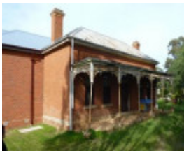
West elevation, 1890s.
