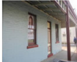
Detail of south elevation.
