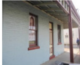
Detail of south elevation.
