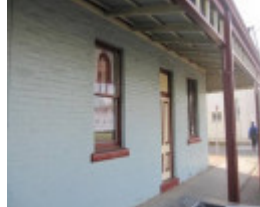
Detail of south elevation.
