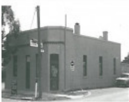
South and east elevations, Lockwood Road and Dunlop Lane respectively, c. 1980s (Source: Ruth Hopkins, Moving Forward, Looking Back: the History of the Marong Shire , 1985, p. 59).
