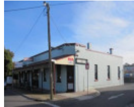
South and east elevations (2010).
