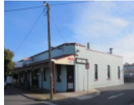
South and east elevations (2010).
