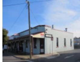
South and east elevations (2010).
